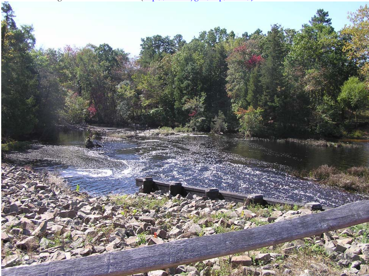
Dam below Batsto Lake, Hammonton, NJ
